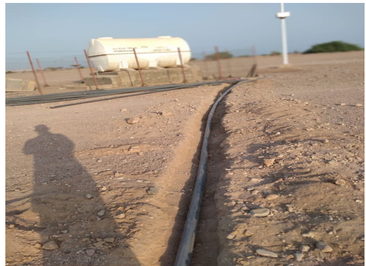
Work Progress of water connection works © Photo: IOM Djibouti 2021
