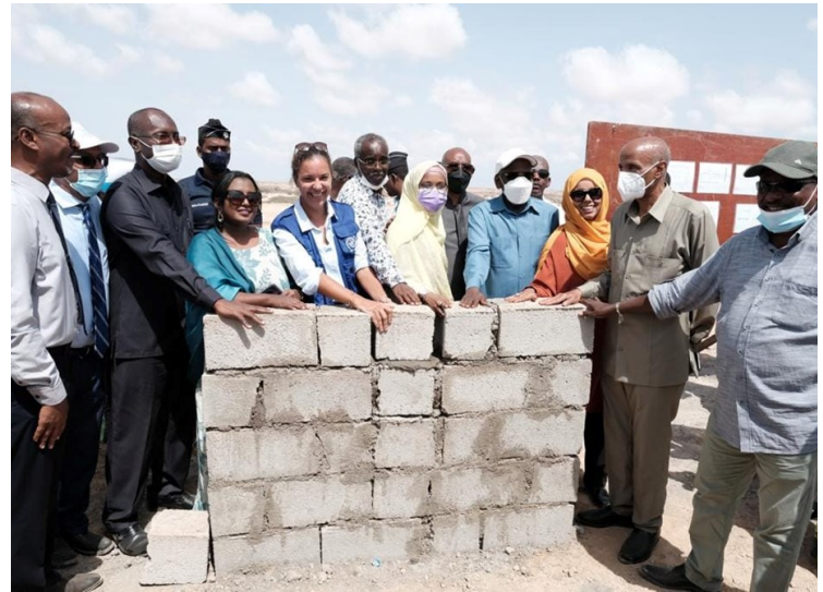
The Prime Minister, accompanied by the delegation, lays the foundation stone of the recycling plant in Obock © Photo: IOM Djibouti 2022
